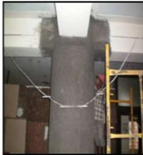
Fig.2.Surface grinded and prepared for fiber wrapping
