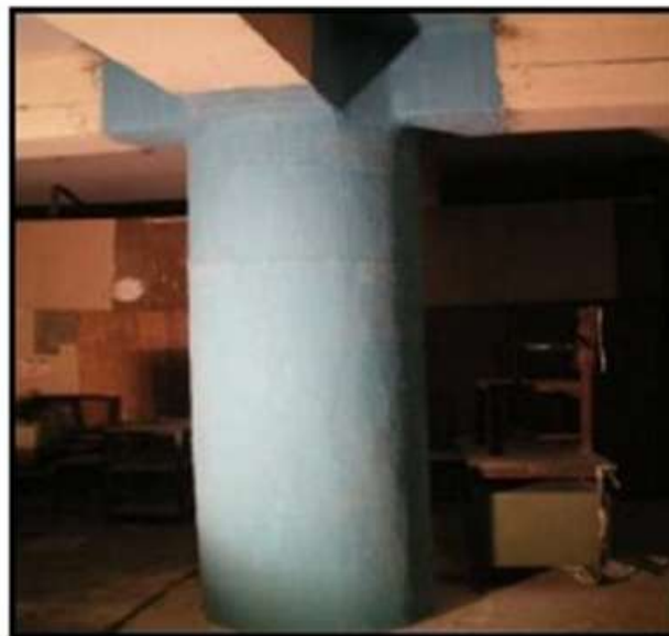
Fig.5.Final look of column after plastering
