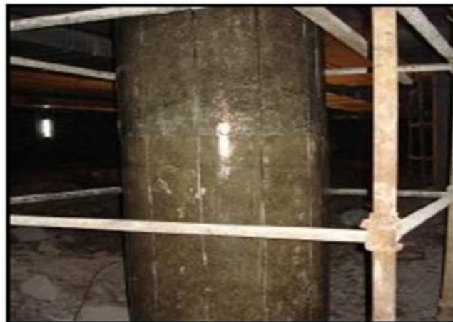
Fig.3.Surface primer applied on the column
