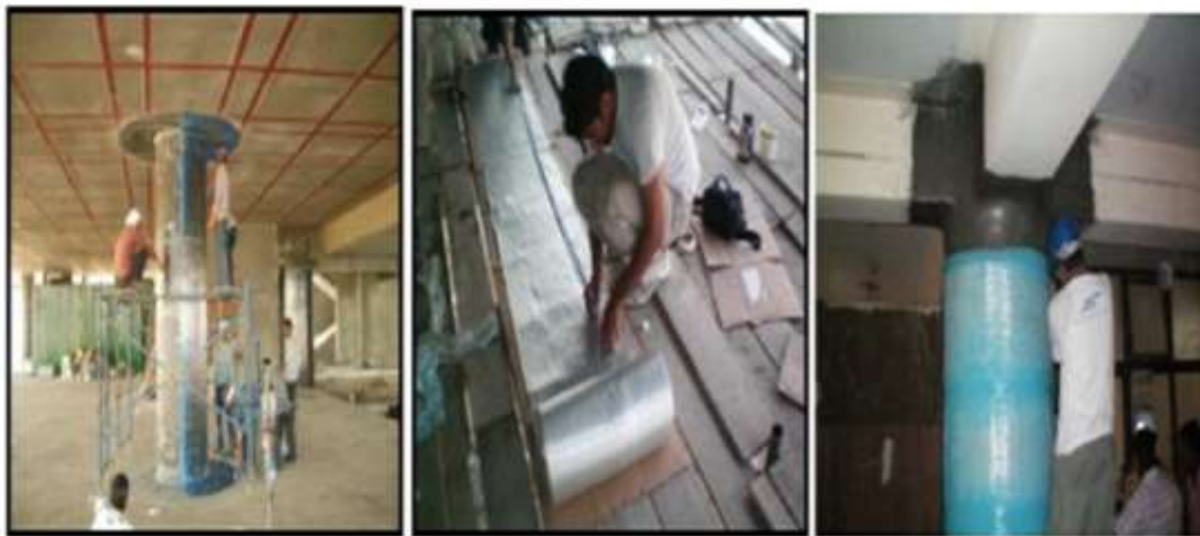
Fig.4.Cutting and applying of fiber sheet on the column
