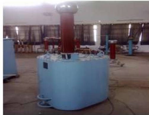
Figure 4. High voltage Testing transformer
