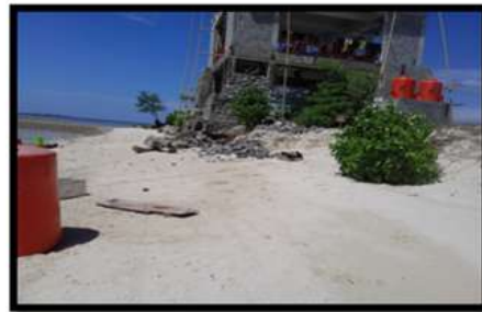
Figure 3 The appearance of homes threatened by abrasion in the eastern part of the island
