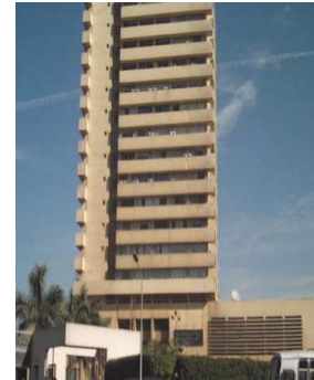
Fig. (2) MWRI Office Complex in Cairo
