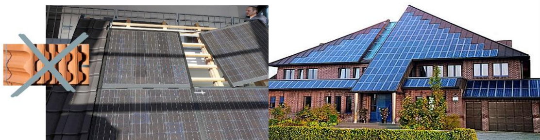
Figure 4: Replacing tiled roofs with solar panels.
