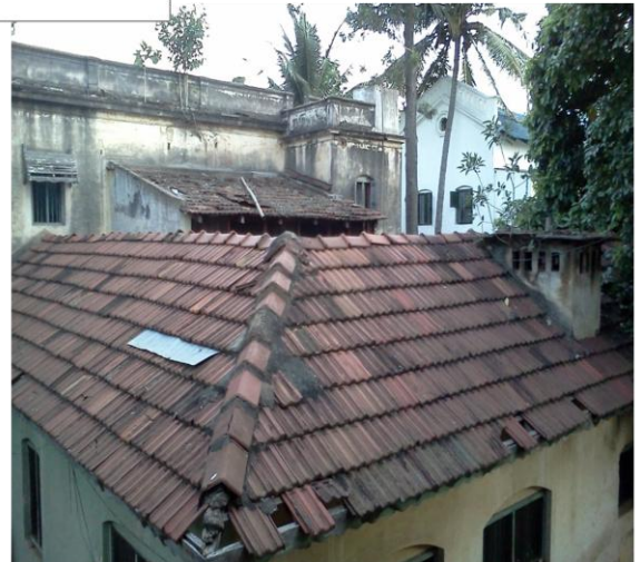
Mangalore tiled with brick walls
