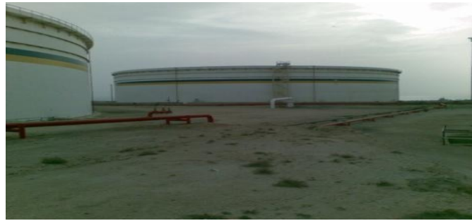
Figure 1- The oil storage tank under consideration in Khark Island
