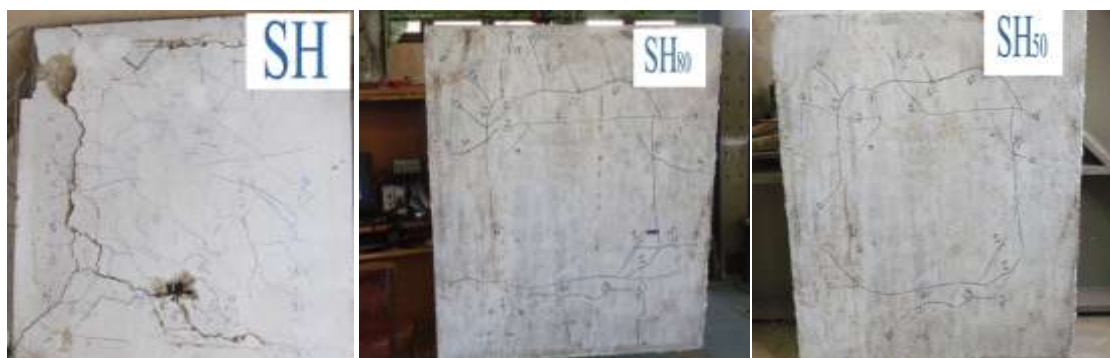
Fig (10): Cracking Pattern for Specimens
