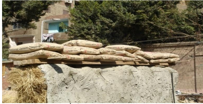
Figure 4: The 2 nd loading case after plastering the wall
