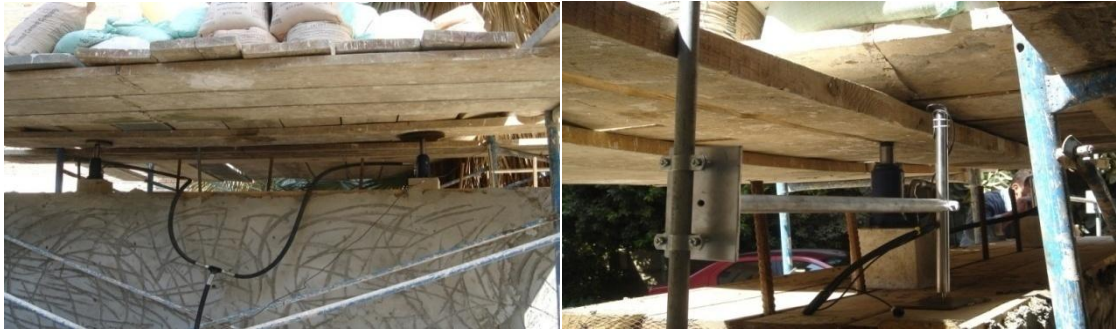
Figure 7: The connection between the Hydraulic Jacks and the LVDTs on Wall B
