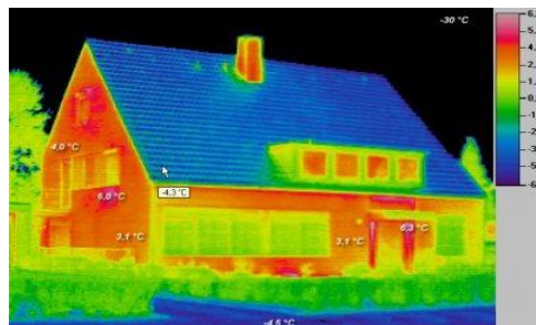
Fig 4: captured image by thermal imaging system
