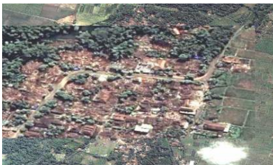
b) After earth quake
