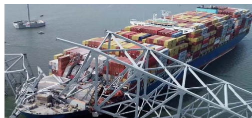
(b) The collapsed Baltimore bridge in USA
