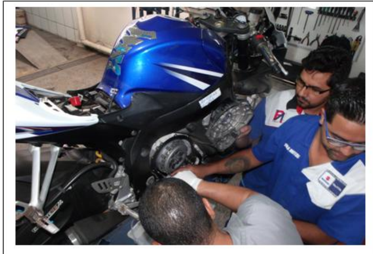
Figure 1 - Engine disassembly by technical Suzuki dealers.
